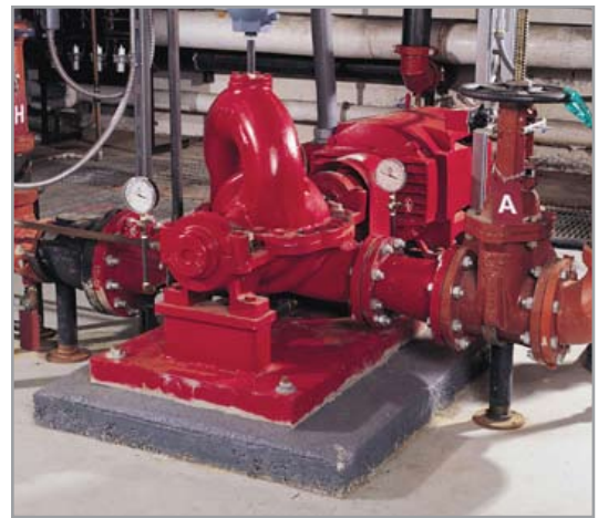
High Pressure Two-Stage DMD Fire Pump.
