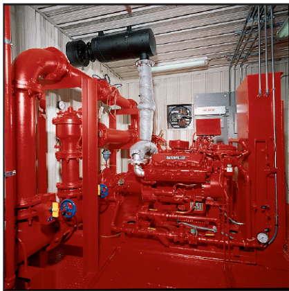
INTERIOR OF A TOTALLY ENCLOSED PRE-PAC.
