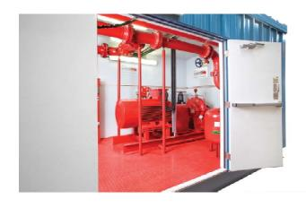
Systems are completely self-contained including suction and discharge lines and valving, pressure sensing lines, test line with flowmeter, fire pumps and drivers, control systems.
