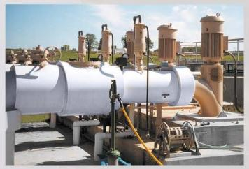
Packing box/tension nut is single piece construction, Type 304 S.S. sleeve over shaft through packing box for ease in assembly and adjustment. Discharge head with high efficiency, continuous radius, miterless elbow and integral splitter vane. The standard line shaft is Type 416 S.S. and is enclosed in a schedule 80 enclosing tube with bronze bearings. Liberal pump column size, resulting in robust mechanical design, which gives favorable
